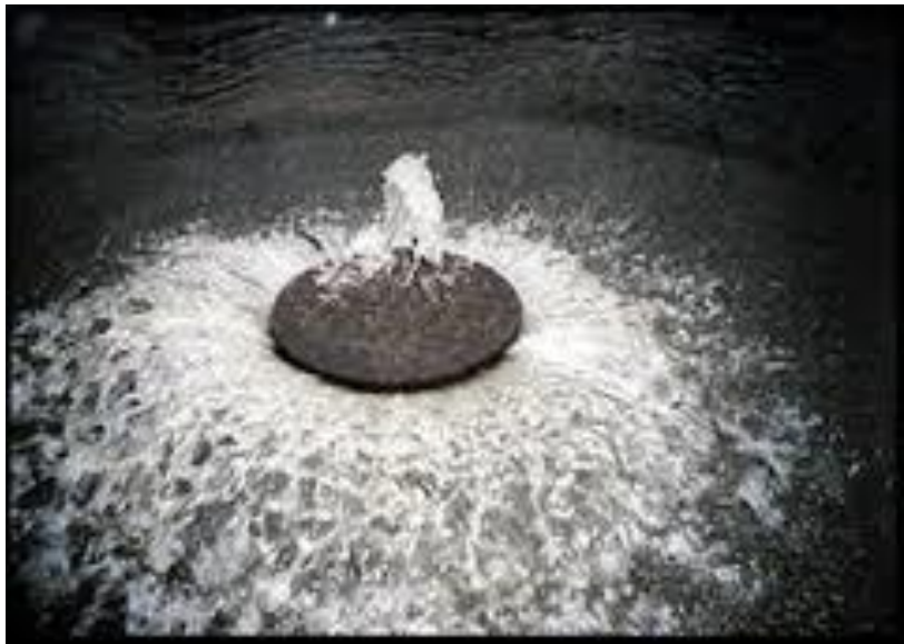
Sewage overflowing into street during a rain storm
