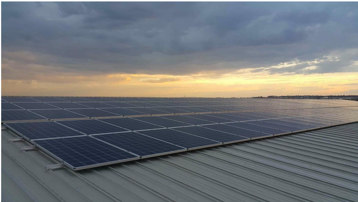
Figure 7.7. Example of Solar PV.
