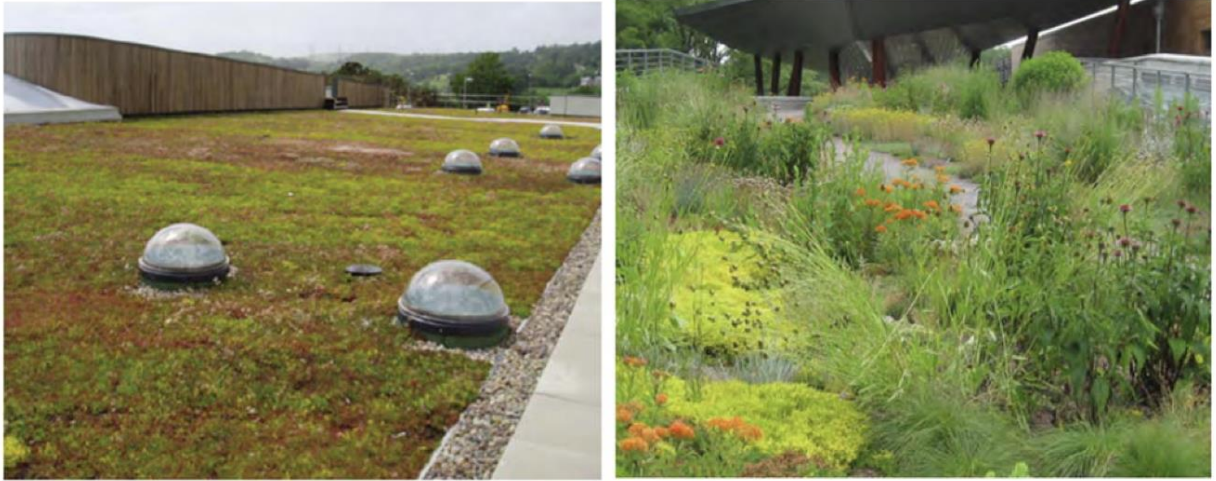
Figure 9.7. Example of extensive green roof (left) and intensive green roof (right) 205
