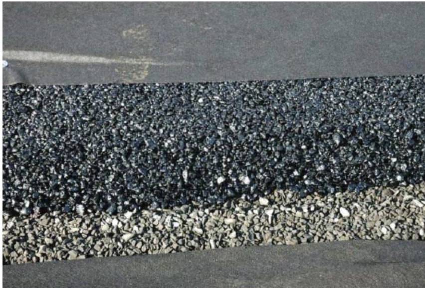
Figure 9.36. Example of porous asphalt pavement. 401
