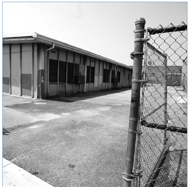
This relocatable classroom or "modular," built with a steel frame on concrete slabs, was supposed to be for temporary use while City Schools await funds for the renovation of the main school building. As of November 2009, 211 moduls are being used by City Schools
