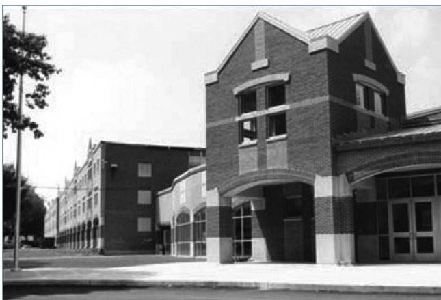
Wilbur Cross High School was completely abated of hazardous materials such as asbestos and reopened in 2002 with wired classrooms, new lighting, a music wing, and expanded library/media center. The new buildings consume on average 30% less energy, which will result in tens of millions saved in utility costs over the next two decades.
