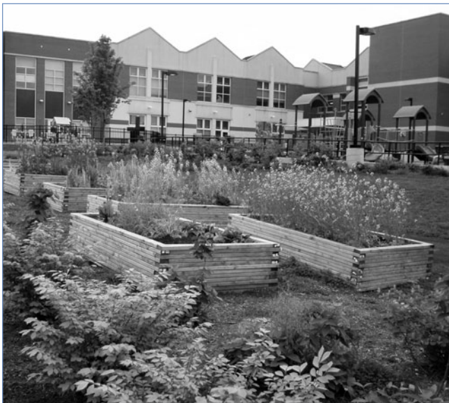
At Barnard Elementary School in Washington, DC, teachers and students worked to install a rain garden to mitigate runoff and enhance the grounds of their newly renovated school. Leaders in Washington, DC, committed to a $3.5 billion school facility modernization plan as part of an aggressive education reform strategy. The new and rehabilitated school buildings bring a sense of renewal into historic communities and neighborhoods burdened with disinvestment.
