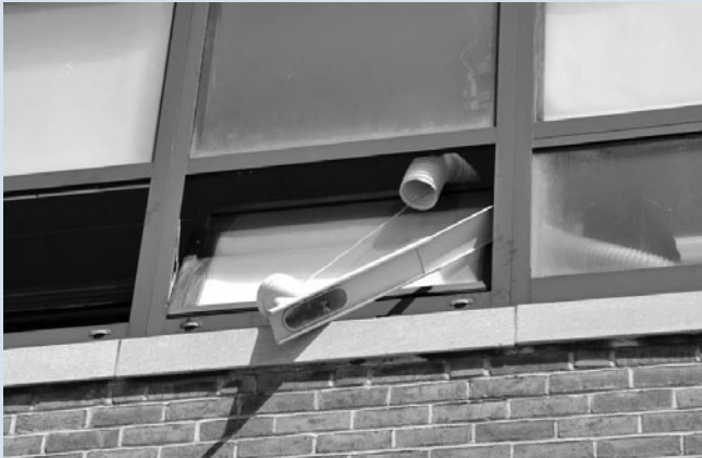
Many city schools have make-shift ventilation systems and air conditioning units. Many windows are broken or do not open. Also, faulty heating systems in schools make some classrooms too hot while others are too cold.
