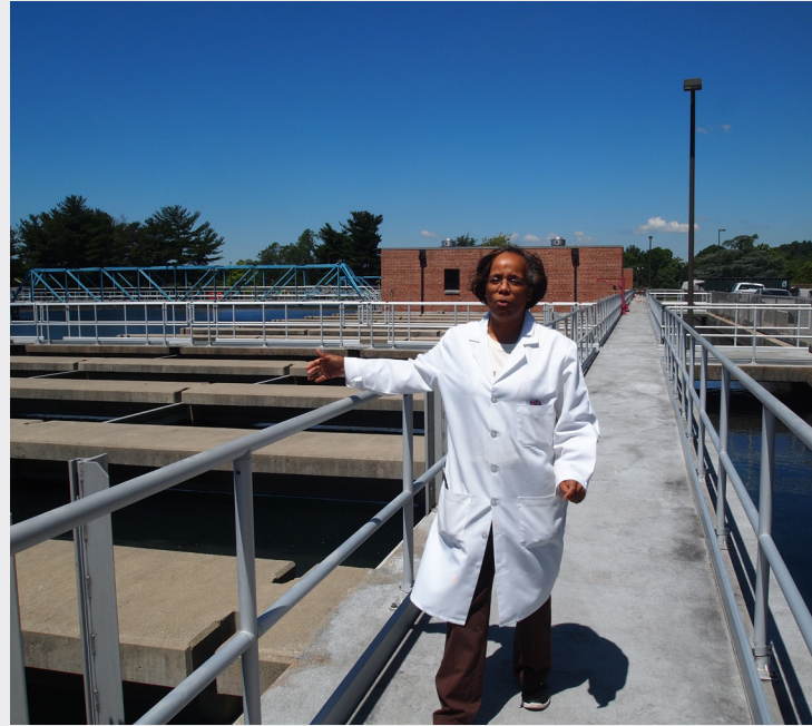
Deneen Gordon, microbiologist at the Ashburton filtration plant in Baltimore, walks through the plant on a recent morning. Photo credit/Rona Kobell
